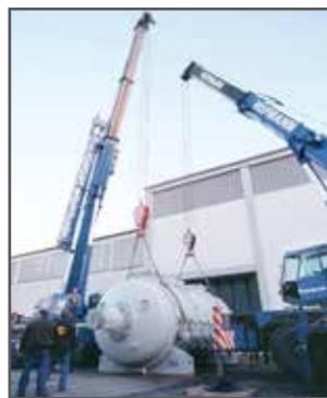
Reactor DVT 55000 while shipment
